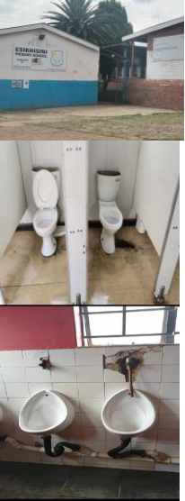
TOILET FACILITY - Before
